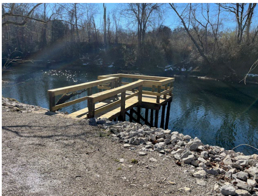
After photo of pier 2 with new decking and safety railing
