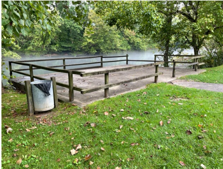
Before photo of concrete pier 3 with spalling surface and failing handrails
