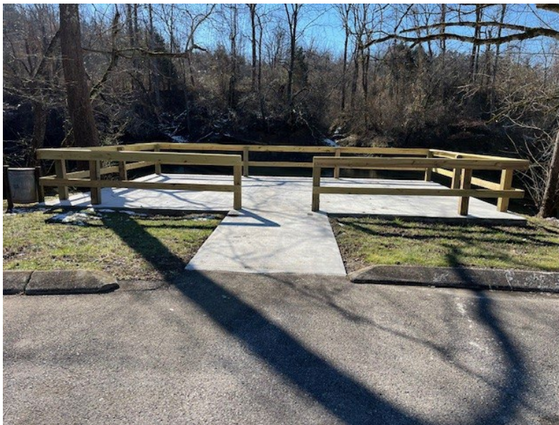
After photo of concrete pier 3 with new concrete surface, safety railing and ADA accessible sidewalk
