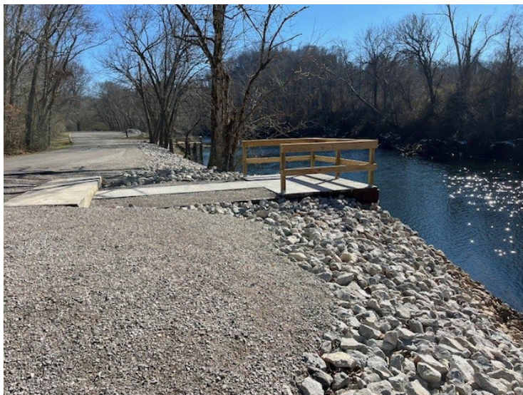
After photo of pier 1 replaced with concrete structure
